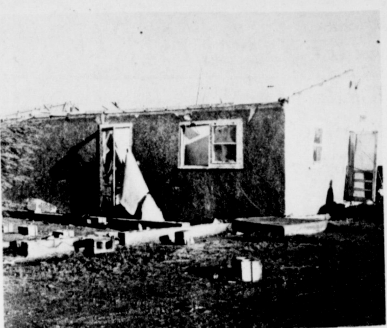
HOME SHIFTED OFF FOUNDATION --This home, behind the Alton Morris farm home east of Lazbuddie, was shifted off the foundation (in the foreground) and demolished in a Friday night tornado. Morris' mother was treated and released at West Plains Memorial Hospital following injuries received in the storm.
