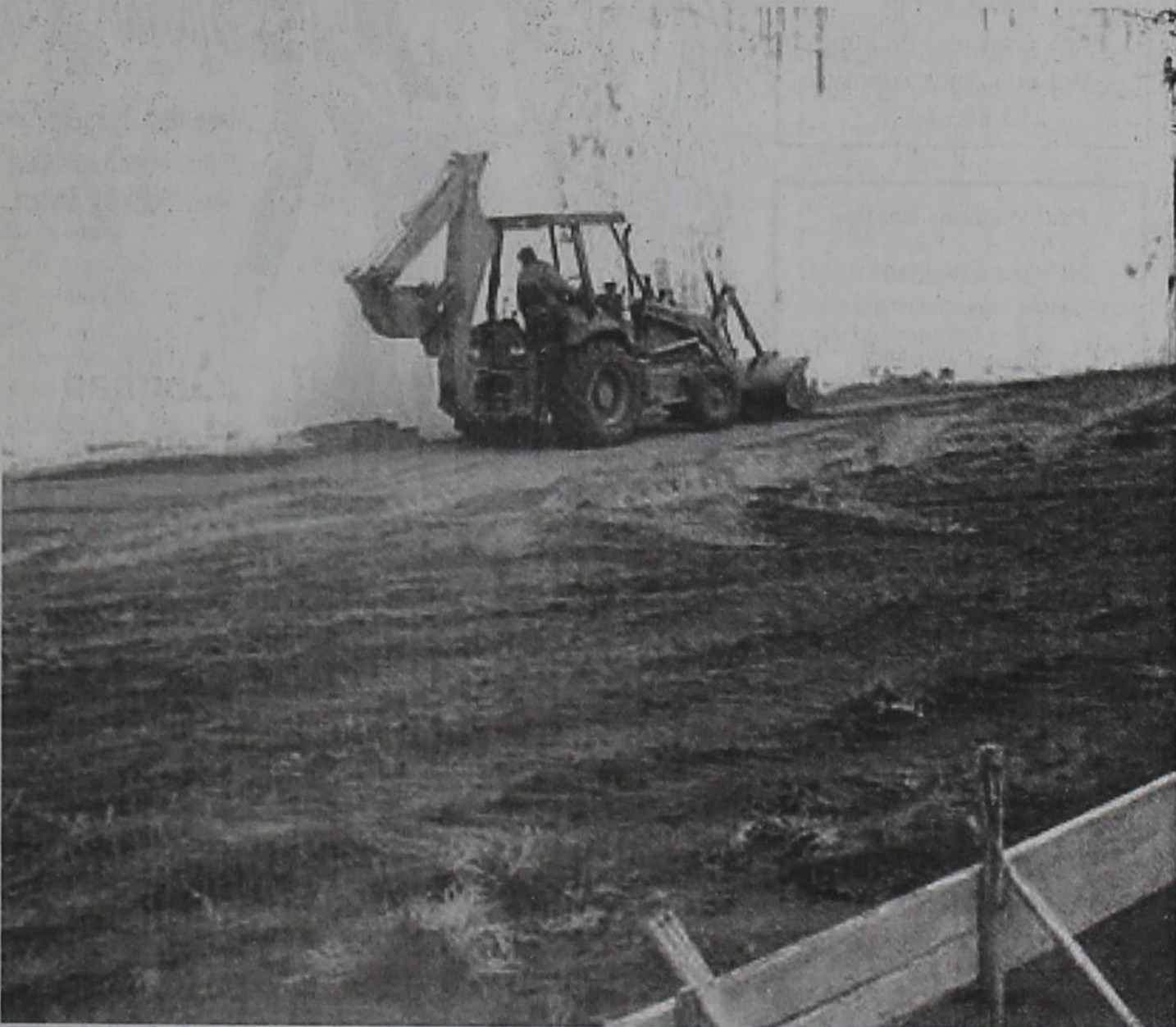
City Crew At Work - Construction Continuing On New Basketball Court
