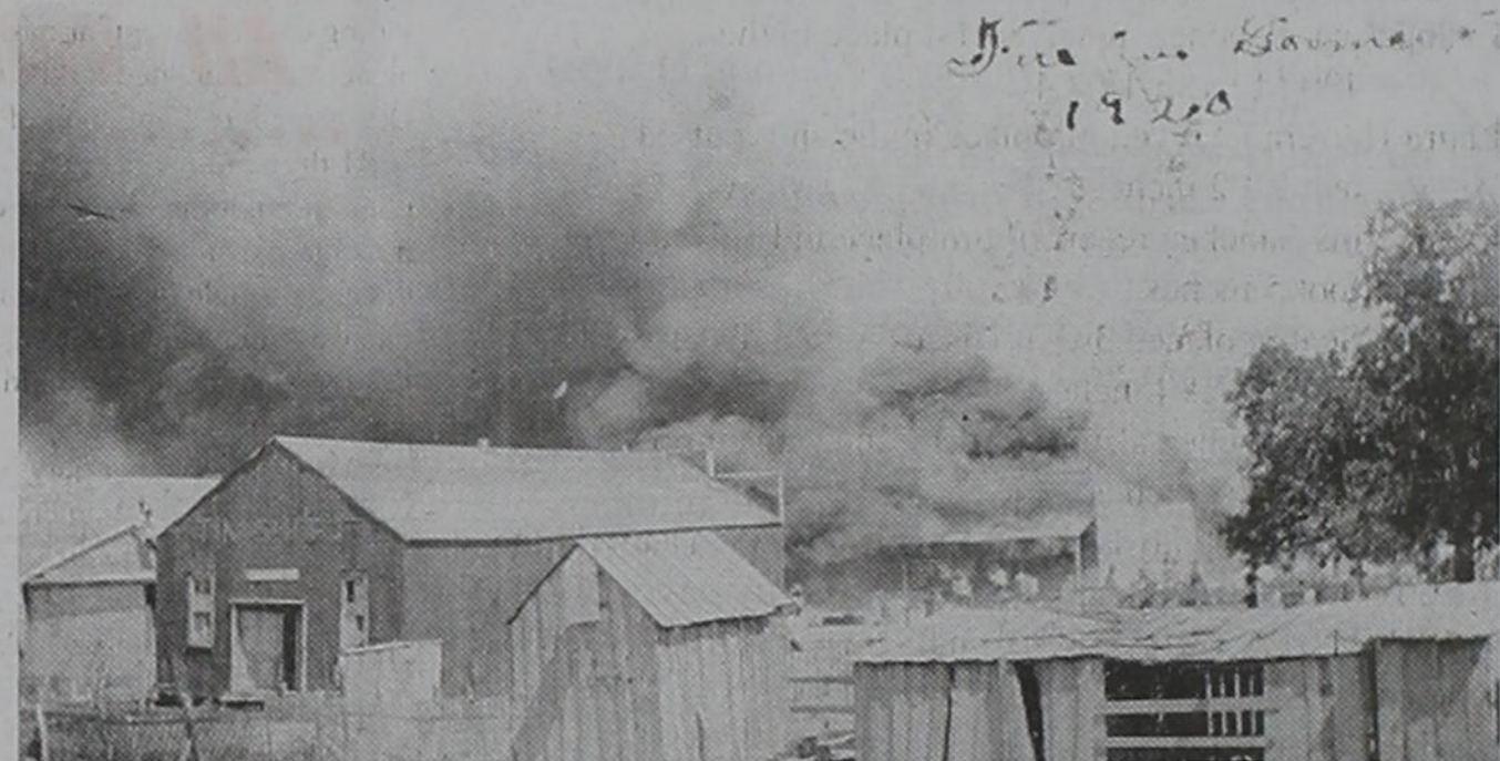
Fire that destroyed commercial block of mostly frame structures across from the water tower, 1920. According to an article in the April 29, 1920 Gorman Progress, the fire caused $100,000 in damage: The Presbyterian Church, Reid & Leatherwood Groceries, Gorman Auto Electric Company, Glass Harper Motor, Mullarky's Garage, Hick's Rubber Company, The Connor Hotel, Kirkley Harness Shop, Cash Grocery & Market, Gorman Bakery, and Gambel Brothers all suffered losses.
