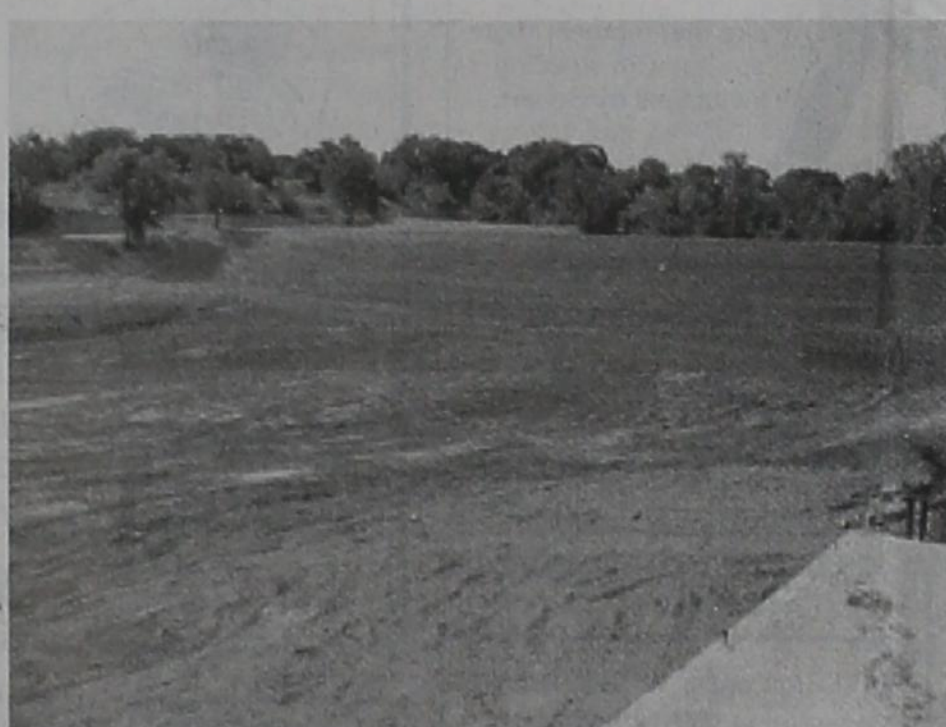
Work on Club Lake Dam completed
