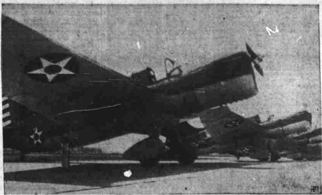
Scout-Observation Planes In Production. Ready for delivery to the U.S. Navy are these seagull (BOGOL) scout observation planes lined up outside the Curtiss-Wright Corporation's Columbus, O., plant. This is the first authorized publication of pictures of the planes designed to serve as "eyes of the fleet." Adaptable to wheels or floats, the seagull can be launched by catapult from cruisers or battle ships.
