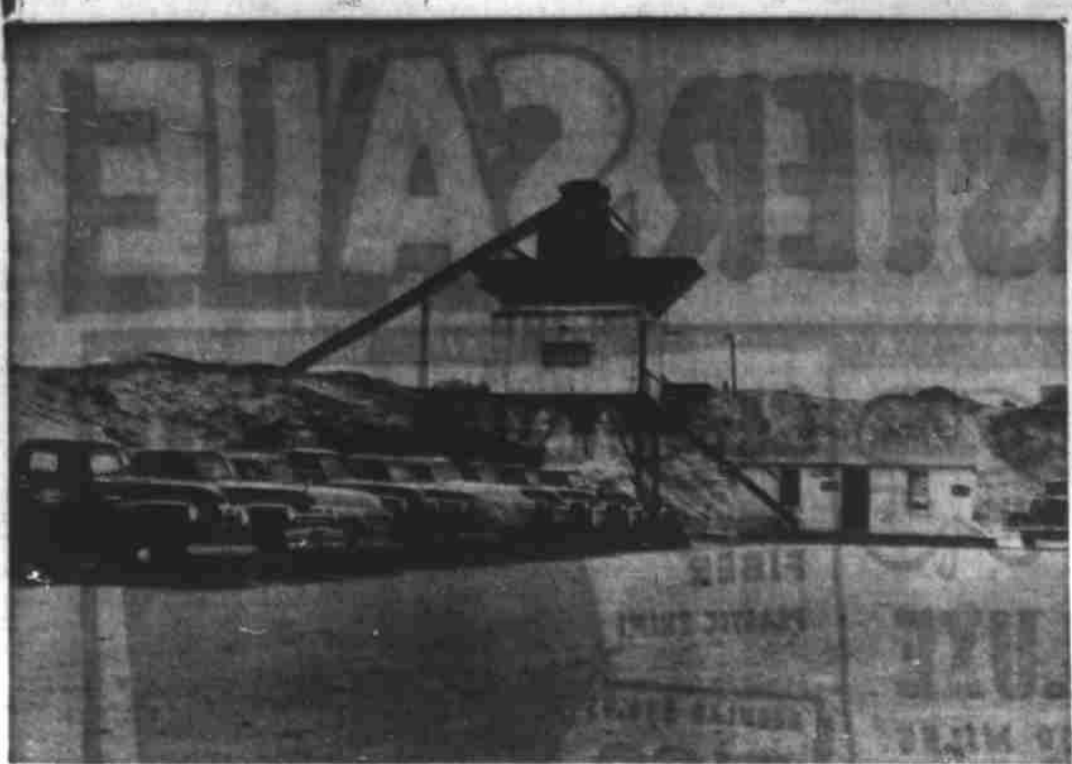
New Concrete Plant
