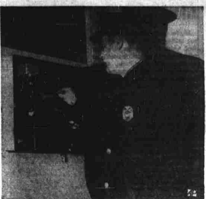
WIRED FOR SOUND —A U. S. Customs guard adjusts the electric-eye alarm apparatus at the guard house on New York's Staten Island, where an intricate system of alarms and signals protects United States' only foreign trade zone. The five pierers of the zone's waterfront are thus protected; even a rowboat entering a slip will sound an alarm in the guard house.
