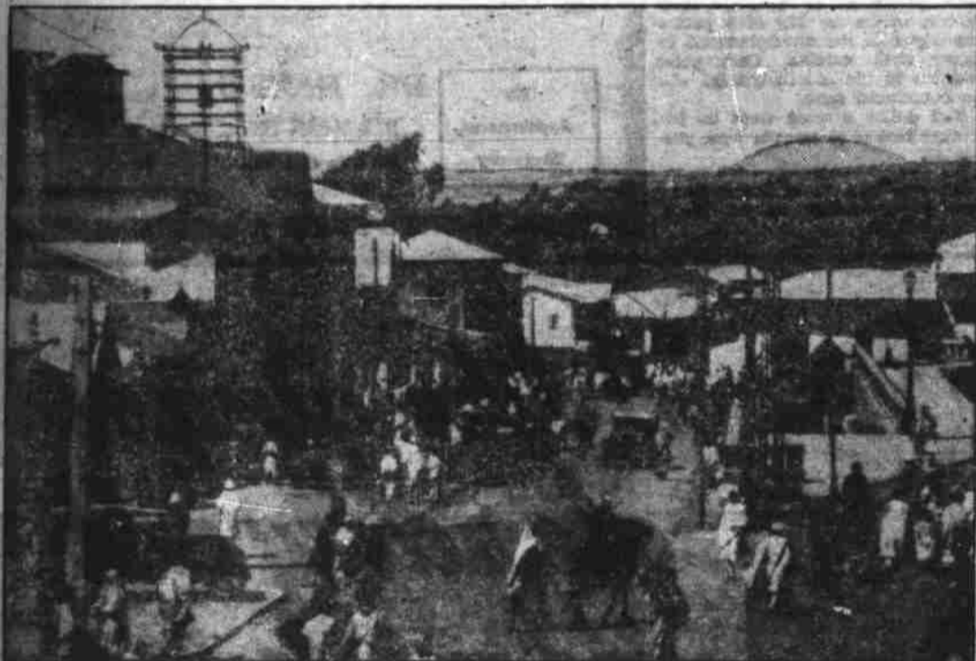
This recent picture of life in Addis Ababa, Ethiopian capital, shows how street activity quickened with the rapid approach of Premier Mussolini's conquering army. The large building at the left is the postoffice, destroyed by marauding native tribesmen. Residents of the capital were preparing bomb-proof shelters when this view was taken, anticipating an Italian bombing raid. (Associated Press Photo)
