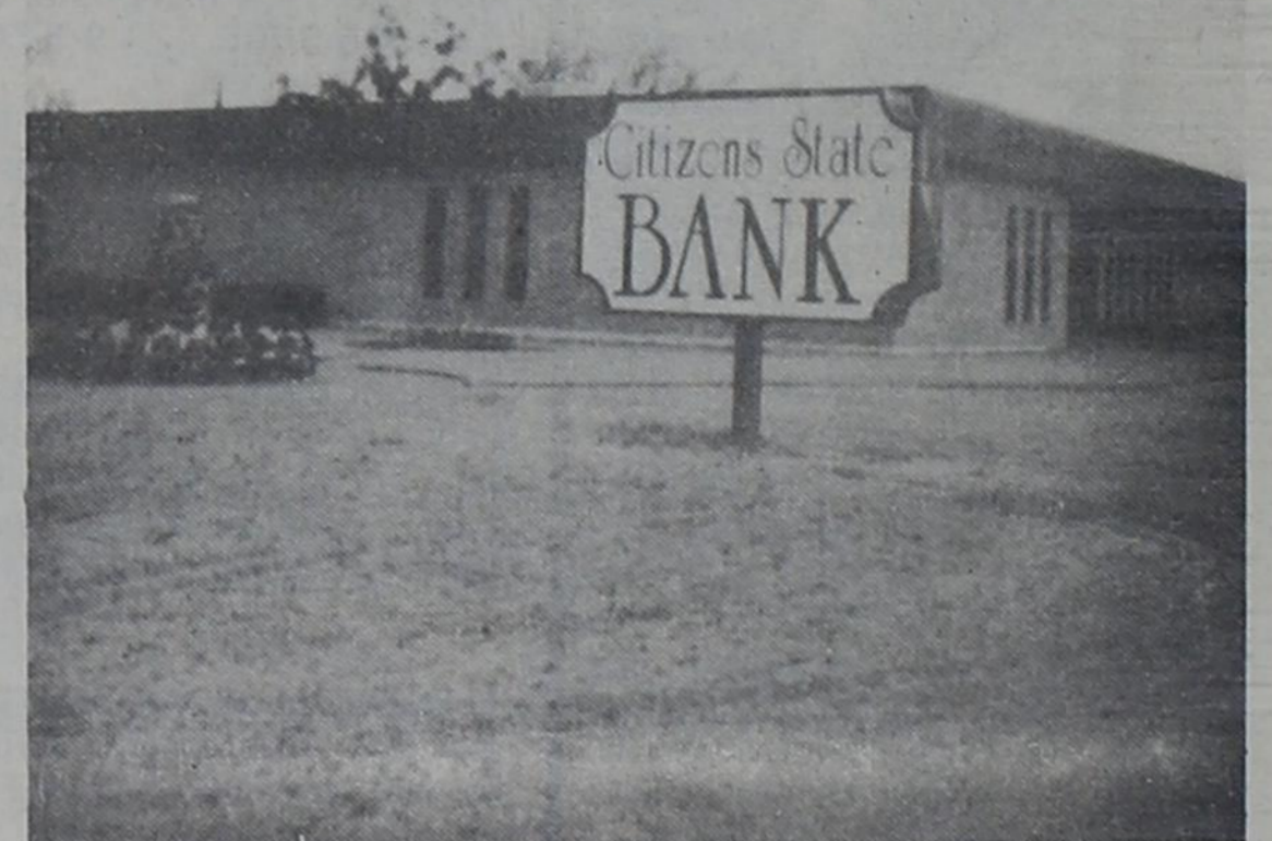
NEW SIGN AT CITIZENS STATE BANK - The new sign shown above was installed Tuesday at the bank. The sign has a beige background with brown lettering.
