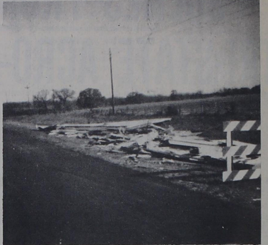
ALL THAT'S LEFT — One half of a Mobile Home was demolished Monday by the high winds, just East of Womack's Nursery on Highway 6. A crew spent most of the afternoon removing the debris from the highway. The truck pulling the mobile home was not damaged when the trailer overturned.
