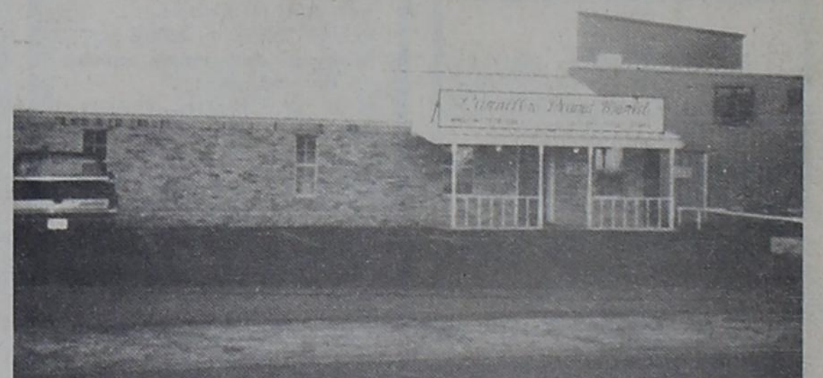
PARNELL'S PEANUT WORLD has completed their new store facilities at their plant on Hwy. 6 West. We hope to have more pictures on this in next week or so.
