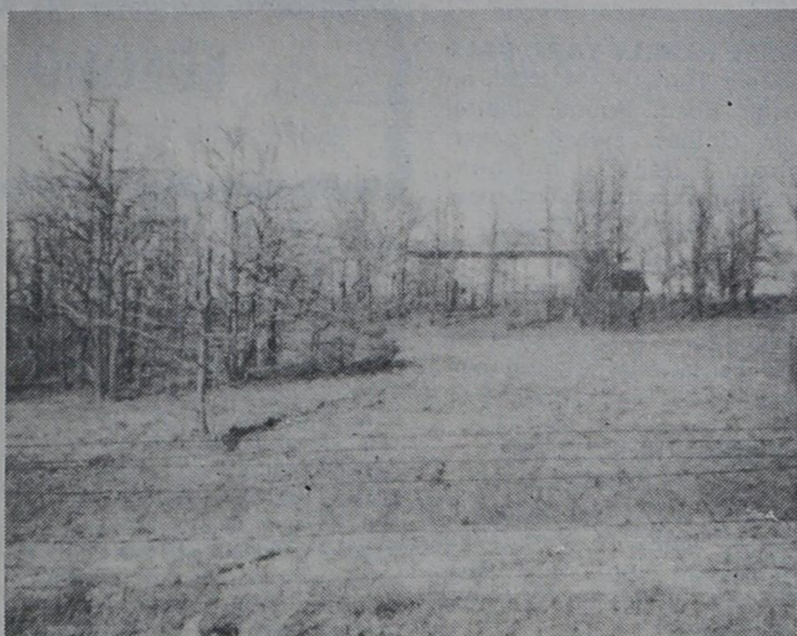
TREES STRIPPED — The trees were stripped all around the home of J. B. Williams out northeast of Kokomo by hail during a severe storm Saturday afternoon. The home also heavy damage as well as other locations in the area.
