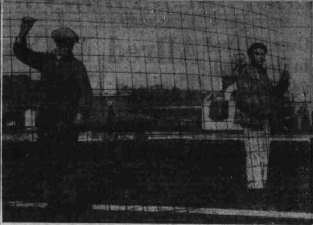
Strength For Heavy Loads—Workmen Tended Steel Mesh In New German "Autobahn"
