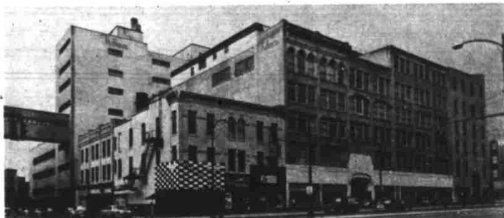
Before the modernization, Thalhimers was a collection of several buildings in this block in Richmond, Va.; the owners decided to cover buildings with aluminum rather than rebuild.
