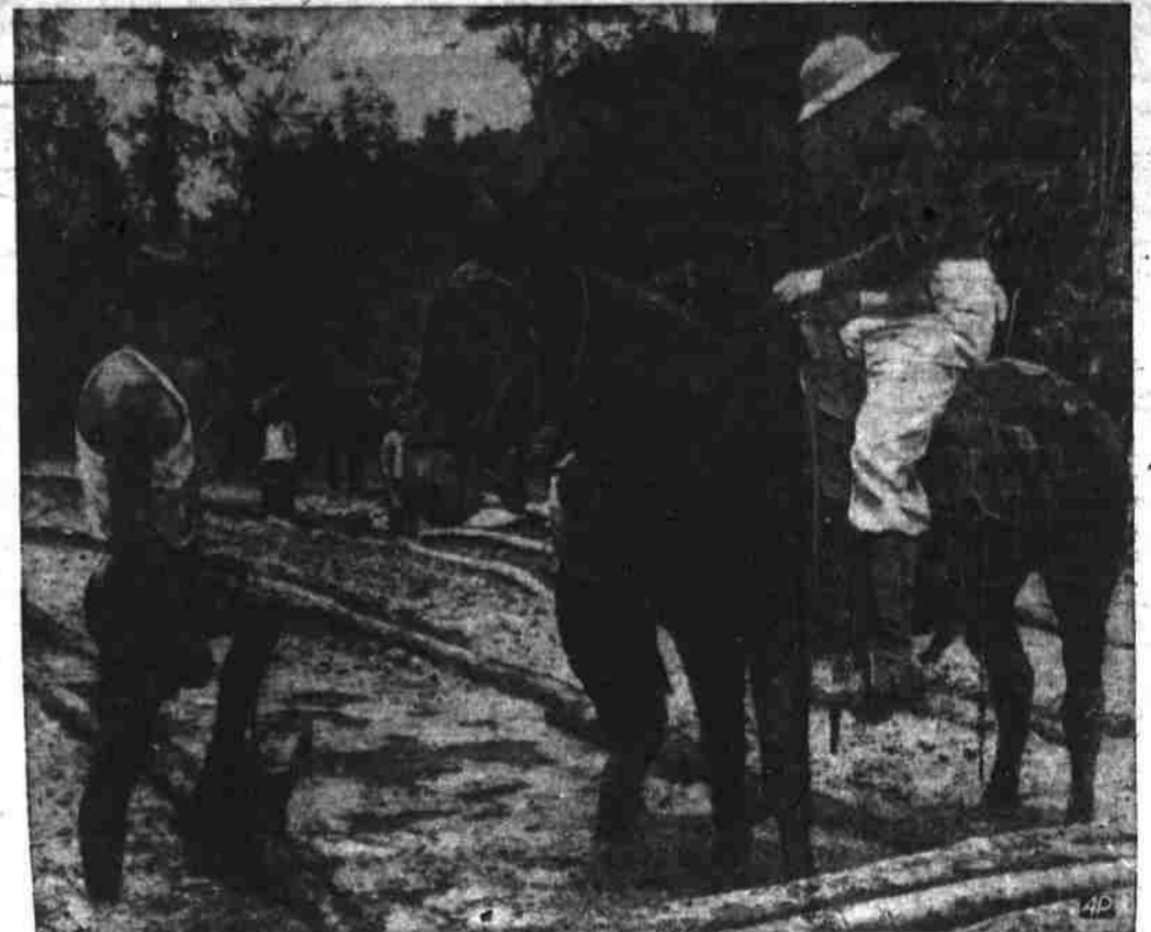
OUT OF MUD AND SLIME —Building stronger defenses for Uncle Sam's vital Panama Canal is a dirty job, as Gen. Sanderford Jarman (on mule) and his men can testify. Jarman, commander of the Panama Separate Coast Artillery Brigade, has been in charge of expeditions pushing through swampy jungles into the Chagres river country to install anti-aircraft batteries.
