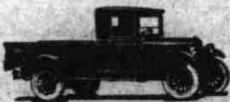
The open express body, with enclosed cab, is widely used by butchers, builders, manufacturers, plumbers—and similar users who do not need to protect the load against the weather.
