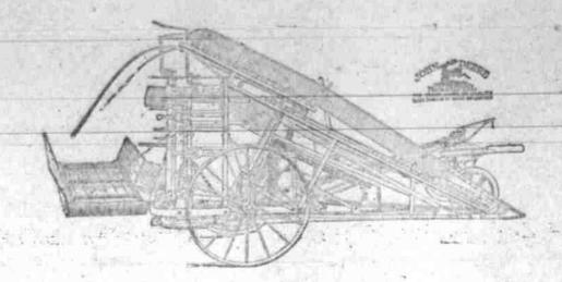
Here is the Binder that will clean up any crop that you ever have to cut. It will bind shorter feed than any machine on the market and will not make your horses necks sore from the weight of the machine as all the weight is taken care of with the new TONGUE TRUCK. Another exclusive JOHN DEERE feature is the POWER BUNDLE CARRIER, which saves you ONE MAN'S time every day you use the machine.
