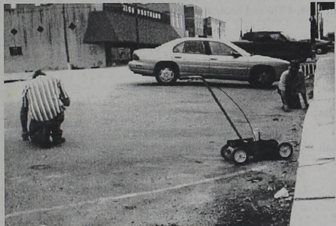
NEW STRIPES — Earlier this month the City Employees were marking and restriping the parking places on Kent Street. The new lines make it easier to park and back out of the spaces.
