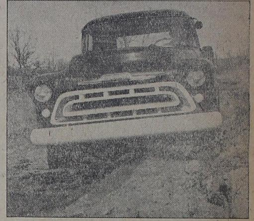
This new four-wheel drive Chevrolet truck plows through hubdeep mud with power and traction to spare. (Note the offset front drive axle under the bumper at the left.) Designed for difficult off-road operations on 1 cep grades, rough terrain, and in deep sand and mud, this all-wheel drive unit now is in production. It is available in 12 models including the suburban carryall; 1/2-ton, 34-ton and 1-ton pickup; 1-ton panel; 34-ton and 1-ton stake
