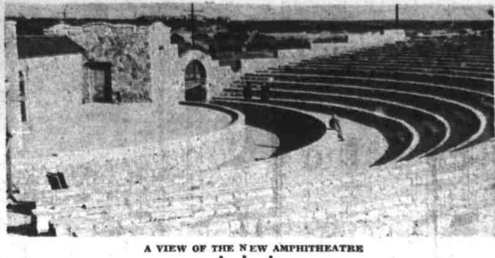
A VIEW OF THE NEW AMPHITHEATRE
