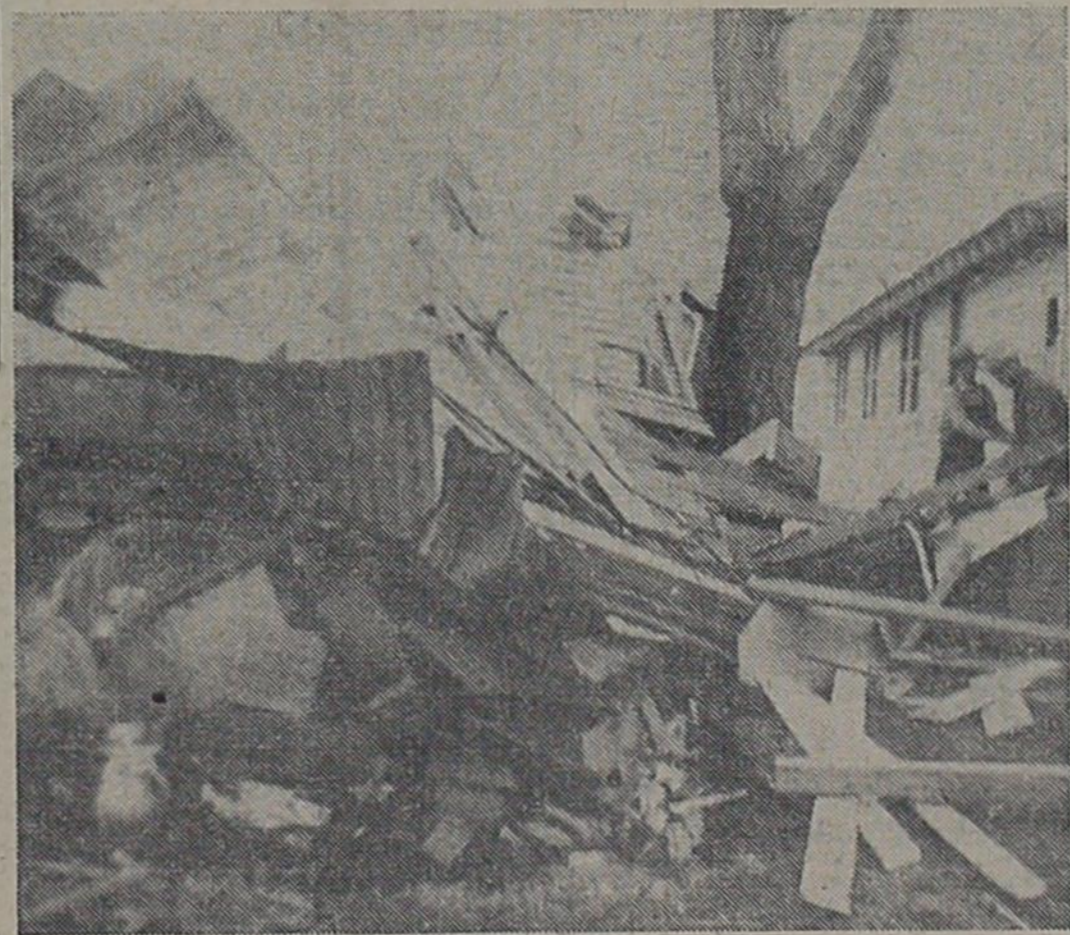
Remains of City Garage after storm Friday, February 19, 1954
