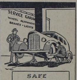
FREQUENT INSPECTION AND ADJUST-ENT OF STEERING GEAR, BRAKES AND OTHER SAFETY DEVICES
