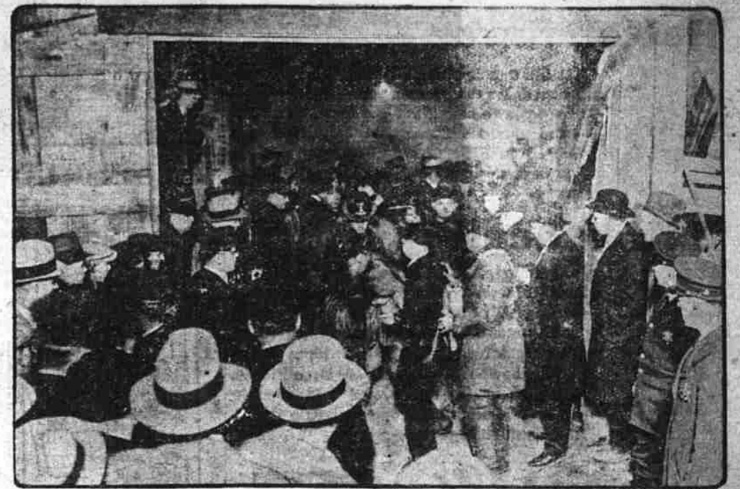
One of the victims being carried out the entrance of a tunnel project on Chicago's west side, where 10 men died and 17 others were overcome by smoke when they were trapped by a fire of unknown origin.
