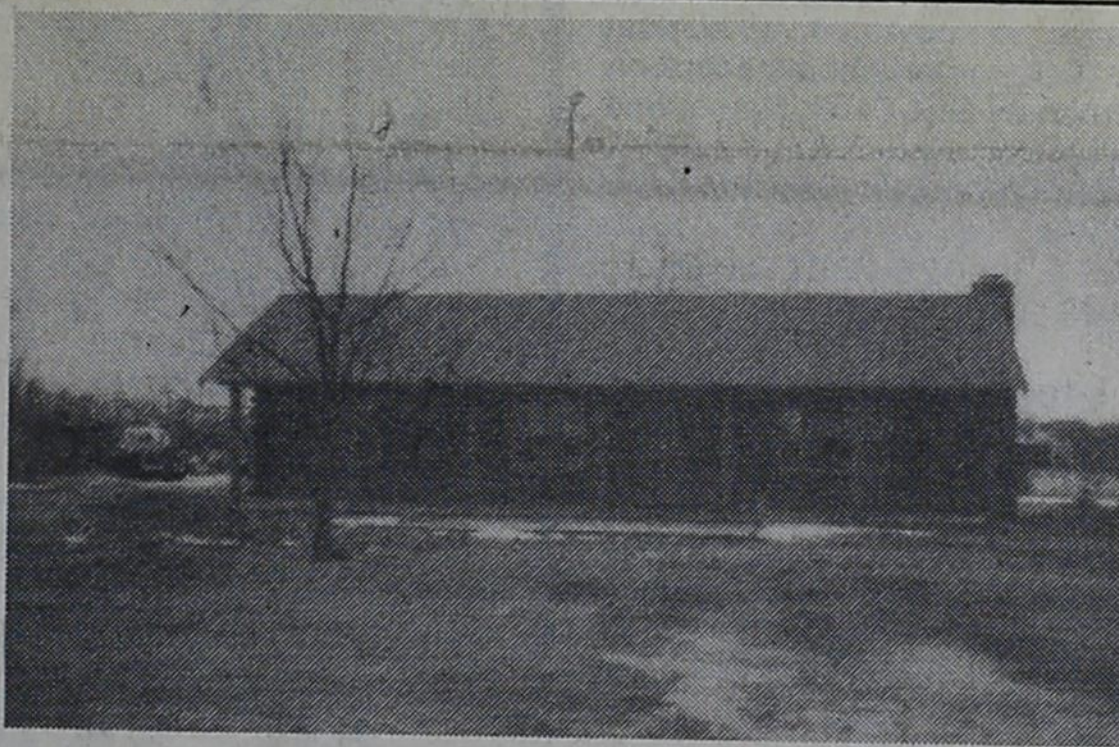
NEW LOG HOME FOR THE A. O. EASLEY'S — Shown above is the recently completed new log cabin home built for the Easleys on the lot west of their office. James Kinser was the builder on the project.
