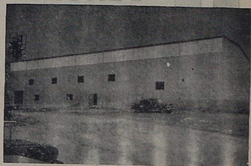
SHELLING PLANT BUILDING — This very large building will house the shelling plant, picking and sacking facilities of Gorman Peanut Company. It is a very large building.
