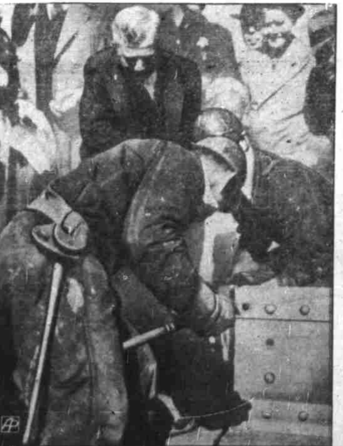
After much ceremony and speechmaking, Ed Stanley (foreground), who drove the first rivet in the Golden Gate bridge, drives home a $400 gold rivet—scheduled to be the last in the huge span—but the head—and the remainder—shattered and fell into the bay far below. A steel rivet was finally used to finish the job.
