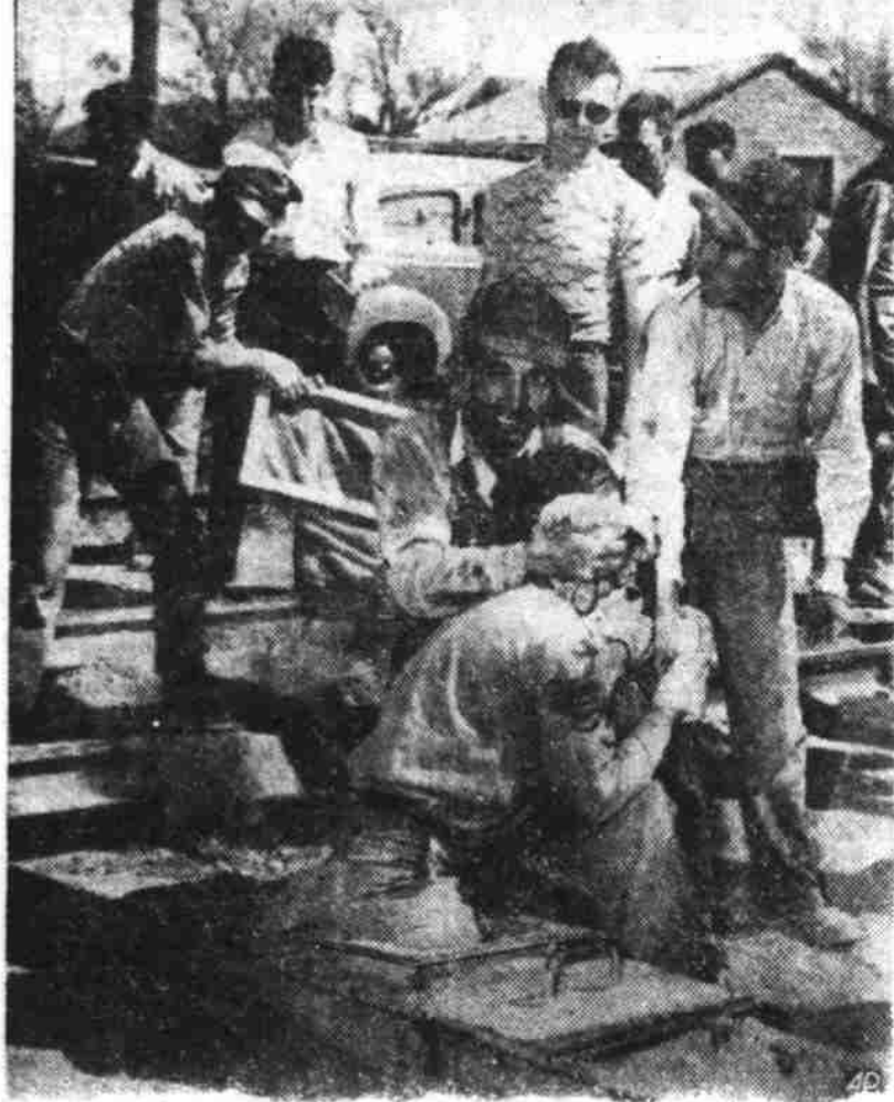
LOSES LEG IN ACCIDENT — Robert Earl Searcy, Jr., Amarillo, Texas, workman who lost his balance while mixing cement and fell, clings to a fellow worker as he awaits help in extricating him from a cement-auger. Welders worked with acetylene torch for thirty minutes to cut the auger and free him. Searcy was taken to a hospital where his leg was amputated at the knee. (AP Photo)
