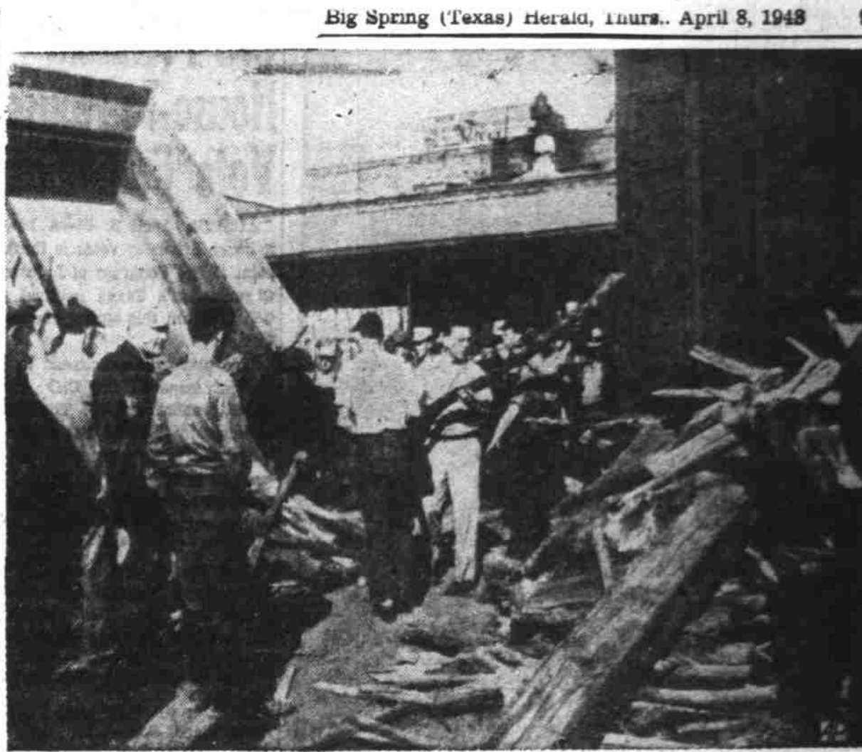
STRIKERS BLOCKADE TRACKS — Striking members of the United Packinghouse Workers (CIO) pile logs and railroad ties on a track leading from the John Morrell packing plant at Ottumwa, Iowa, in an effort to stop removal of meat from the plant.
