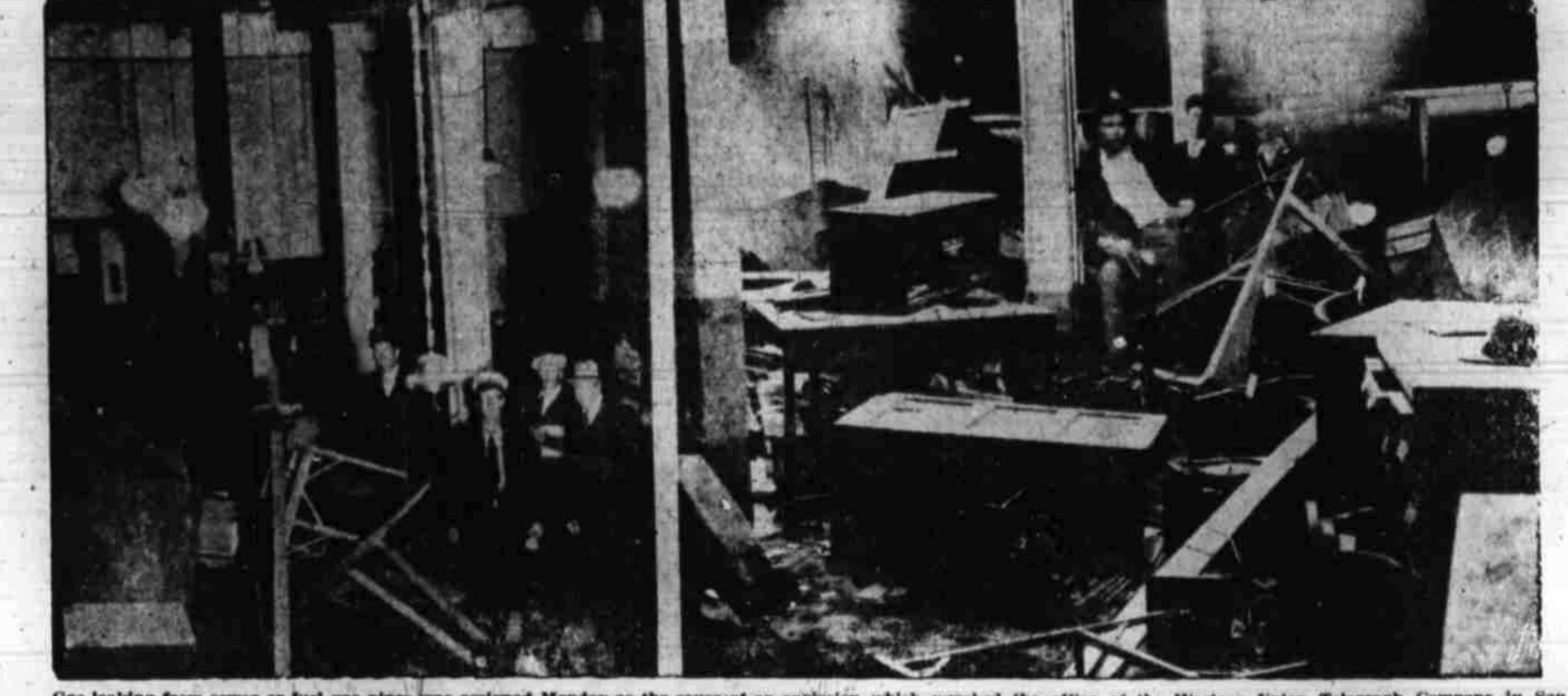
Gas leaking from sewer or fuel gas pipes was assigned Monday as the cause of an explosion which wrecked the office of the Western Union Telegraph Company in San Angelo Saturday evening. The pictures above show the effect of the explosion, which injured seven persons, two seriously enough to be confined in hospitals. Fire Chief John Parker, in the center of the picture, wearing a white cap, at first advanced the theory dynamite might have caused the blast.
