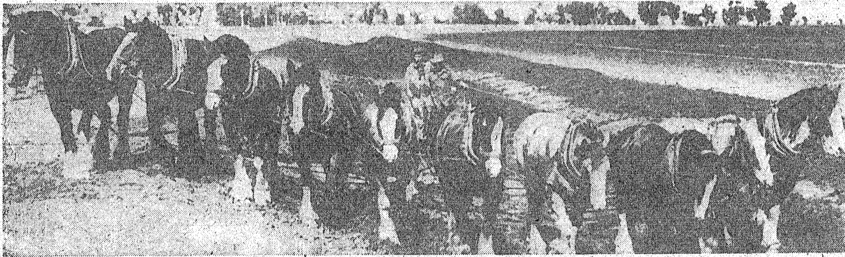
TEN HORSEPOWER DIGGER IN ACTION —In these days of power-driven machinery, a ten-horse team is a rare sight even in Australia. This ten-horse team is at use in building an irrigation canal in the Murray Valley soldier settlement near Victoria, Australia, where between 500 and 600 miles of irrigation channels are being excavated. Horses are being used in moving the dirt in preference to motor-driven machines because the stamping of the horses' feet helps bind the soil on the banks of the irrigation canals and thus prevent water erosion. The horses are worked all abreast instead of being strung out in five pairs as is customary in this country.
