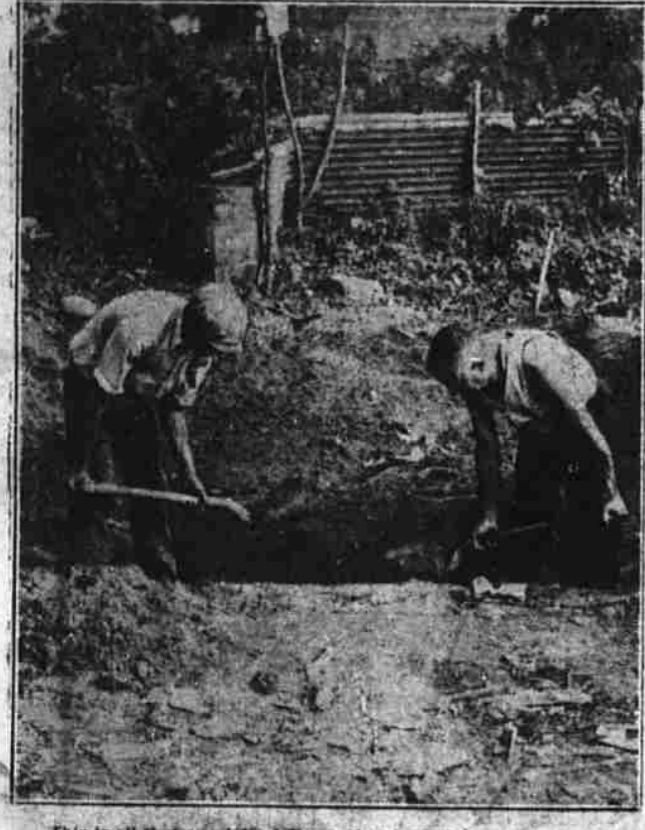
This is all that was left of Bruno Hauptmann's garage in the Bronx, New York, after Lindbergh ransom investigators had dismantled it in their search for further clues in the case. Workmen are shown digging around its foundation. The daughter of Hauptmann's landlady said the suspect had built the garage himself, and had installed an elaborate alarm system connected with his bedroom. (Associated Press Photo)
