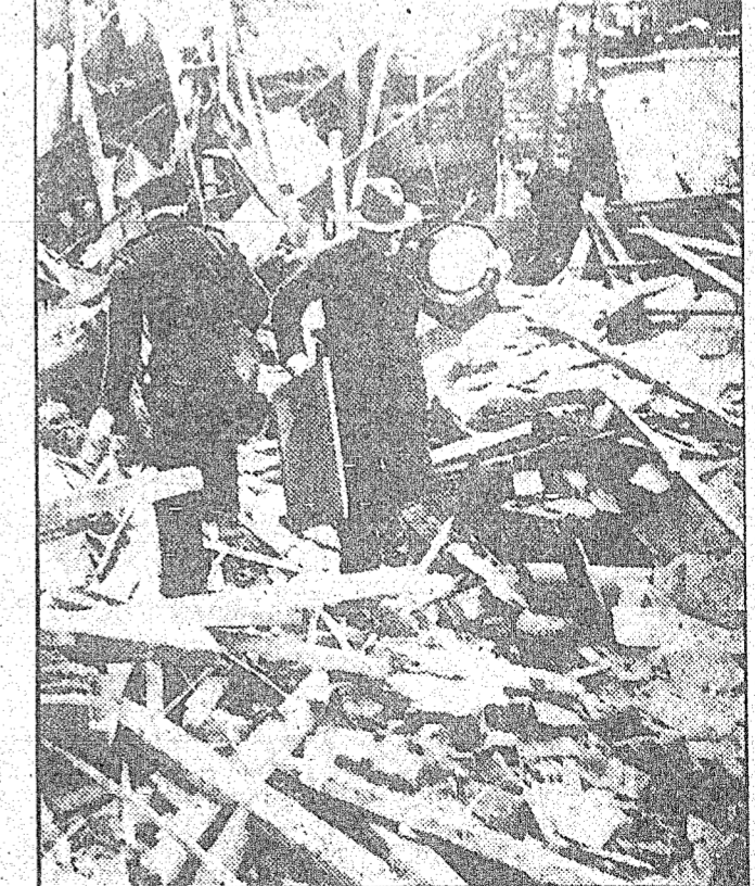
WHEN BOMBS wrecked his home, this London householder salvaged a clock and some of his furniture. German bombers ruined the residential area in a recent raid.
