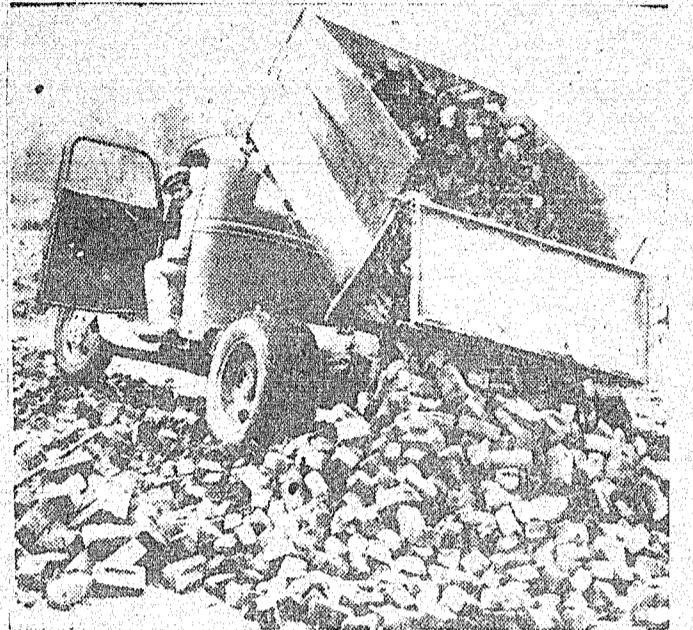
LONDON TO HOUSTON —Brought to this country as ballast aboard a British freighter, bricks from bomb-torn London become part of Houston, Texas, highway. They'll serve as road foundation.
