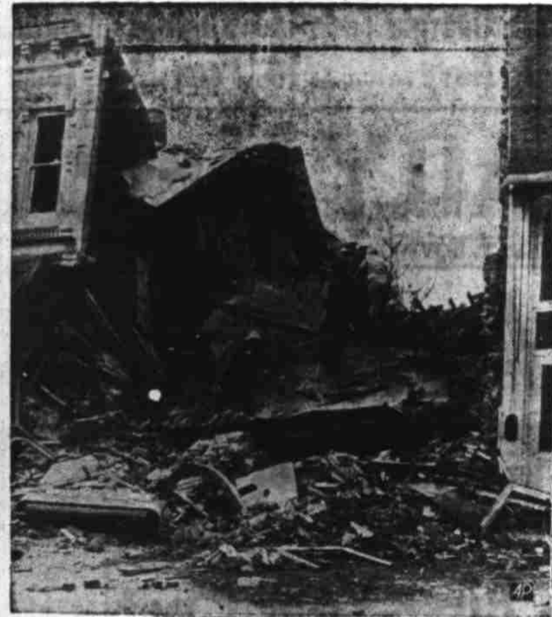
TWO INJURED IN EXPLOSION — Debris marks the spot where the Oregon Electric Shop stood in Oregon, Mo., before an explosion wrecked the building, critically injuring two persons. The office building at left is just a sagging wreck while the grocery building at right was severely damaged. (AP Wirephoto).
