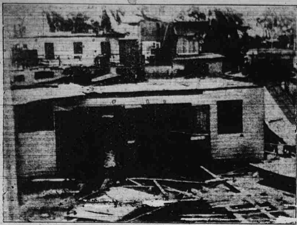
This Associated Press telephoto shows some of the wreckage in Hato Rey, suburb of San Juan, Puerto Rico after the hurricane which killed 212 persons, injured more than 2,000 and left 245,000 homeless.
