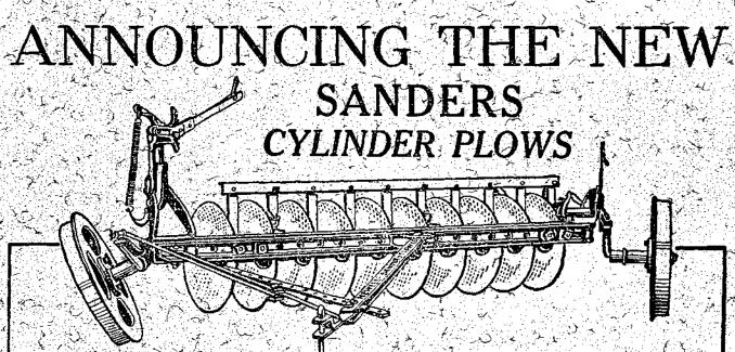
Large Capacity. Light Draft. A general purpose plow. Ideal for Summer plowing but equally good in Cotton, Corn and Maize in the Pall. Plows 2 to 6 inches deep. Easily adjusted and operated. Turns the soil over: Leaves the surface theroughly harrowed and without ridges.
