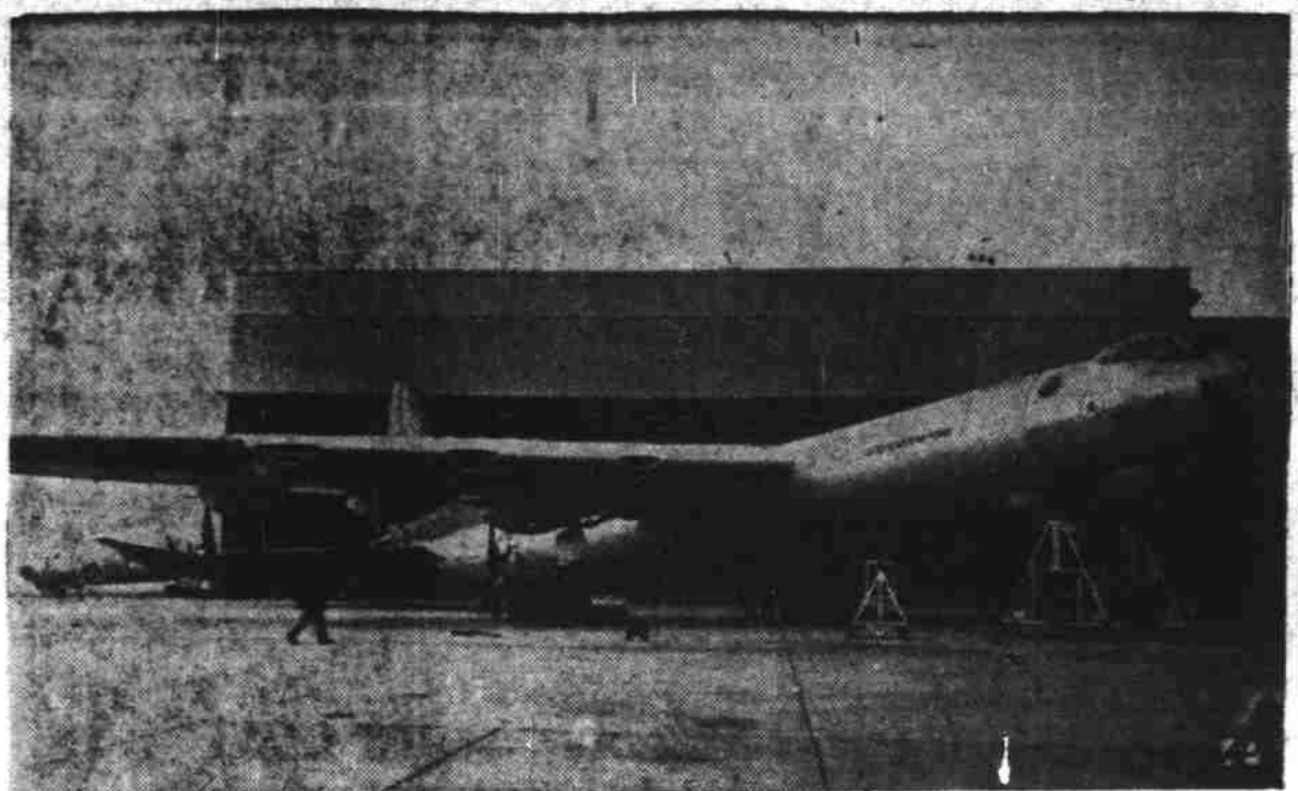
NOSE HIGH - Getting the world's largest bomber out of Consolidated Vultee's assembly plant at Fort Worth, is a problem. The 230-foot wingspread won't clear the 200-foot wide door and the 47-foot tail is too high for the door. The solution; turn the B-26 sideways and jack up the nose, which drops the tail. This one has just cleared the doorway. (AP Wirephoto).
