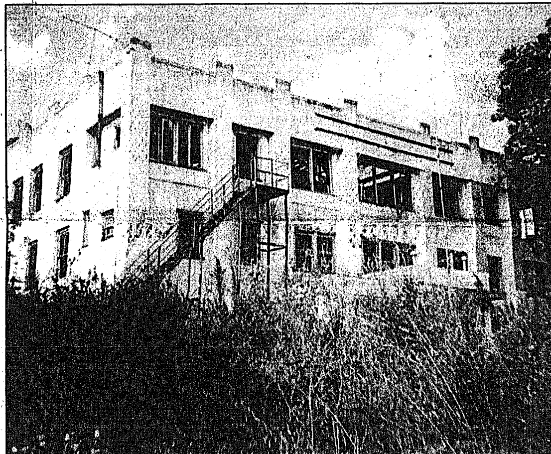
The HDO recommends demolition of Sealy Hospital bldg. after an engineer has advised against trying to restore it. What do you think? Let the HDO know how you feel about it.
