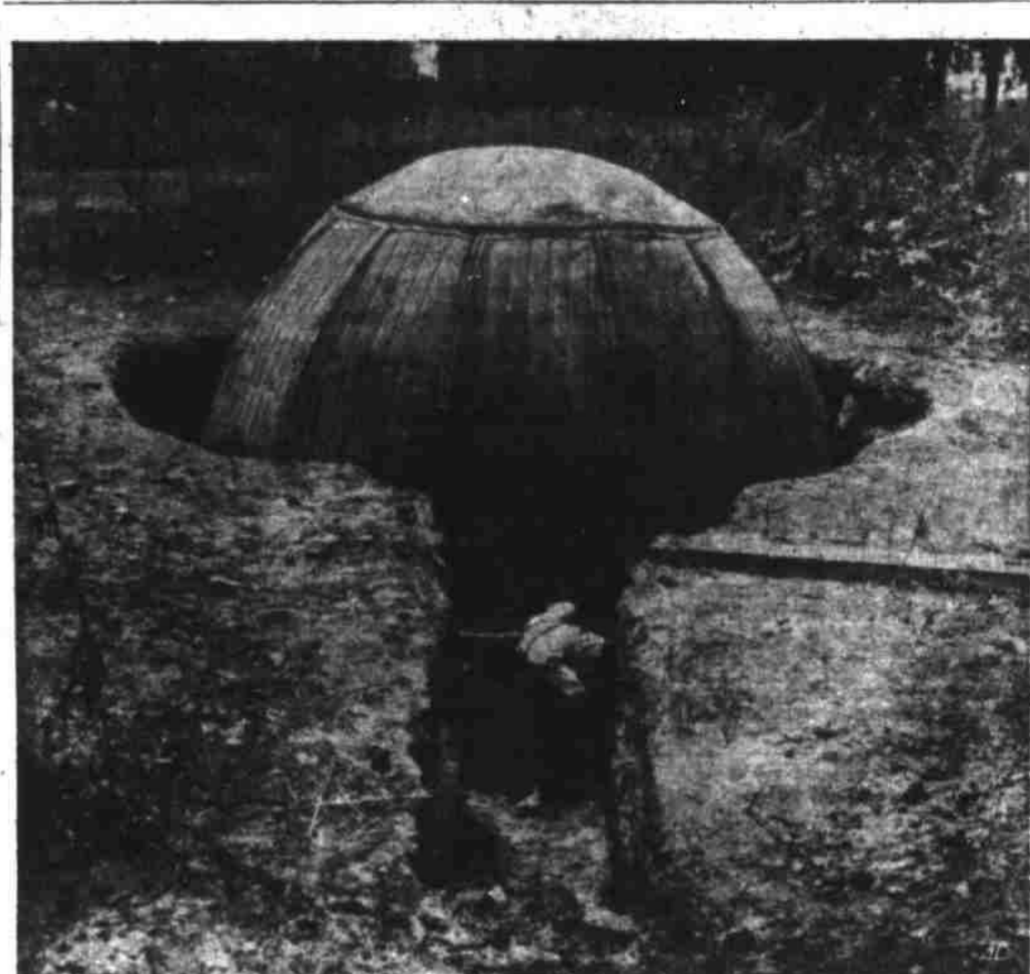
BITTER PILL—FOR AN ENEMY— At least one "John Hubbell" inspects first-hand a bomb-resistant pillbox demonstrated to army and navy leaders in Washington at an isolated spot along the Potomac. Built of concrete in five hours, complete with gun openings and trench approach, the pillbox supported weight of three men a few hours later.
