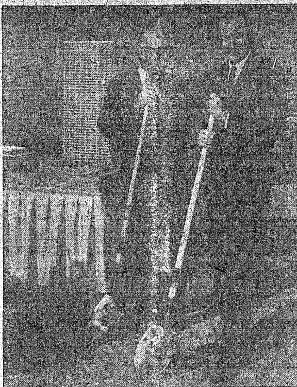
SPADEWORK ON HUMBLE'S NEW HOME — In Houston, Morgan T. Davis (right), president of Humble Oil & Refining Company, turns the first shovel of soil for Humble's new 34-story office building shown in the background model, while Humble Division President Ray H. Horton joins in the ceremony. The 600-foot structure, with some 1,000,000 square feet of usable space, is scheduled for completion in late 1962.
