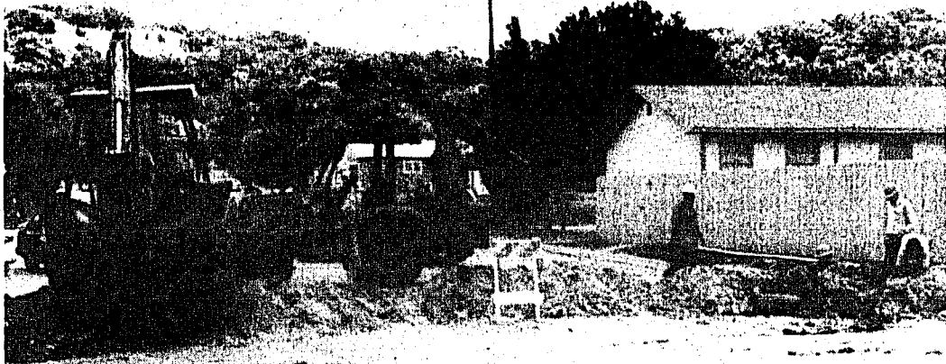
Stewart Construction workers laying conduit for CCTC underground feeder routes.
