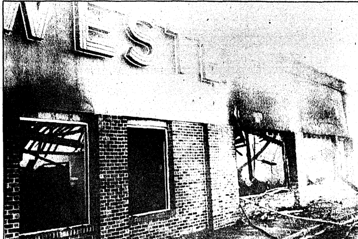
FIRE IN BANGS : The Western Auto Store in Bangs was destroyed by an early morning fire on Tuesday. The Bangs Fire Department responded to the blaze at 4:45 a.m. and battled the blaze at the business located on Kyle Street. The store and its contents were determined to be a total loss. The Artie B Styling Salon on the east side of the store received minimum damage and the Bangs Upholstery on the west side received a bit more. The Brownwood Fire Department and Lake Brownwood Volunteer Fire Department assisted the Bangs firemen with the blaze.
