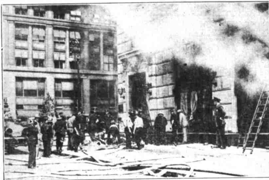
An explosion shook the 42-story Ritz Towers hotel on New York's fashionable Park avenue, killing five firemen and injuring more than 26 persons. The explosion occurred in a paint shop below the street while firemen were fighting a basement fire. The blast smashed the front of a jewelry shop and more than $100,000 in gems were scattered in the street. (Associated Press Photo)
