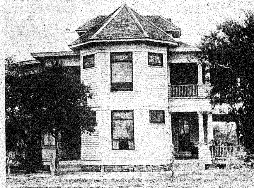
EARLY DAY FINERY. The late J. D. Simpson added bay windows, front rooms and porches with large columns to the original two-story structure, as shown in an early picture of the historic home. Mrs. Kitty Adams is the only family member still living in Santa Anna.
