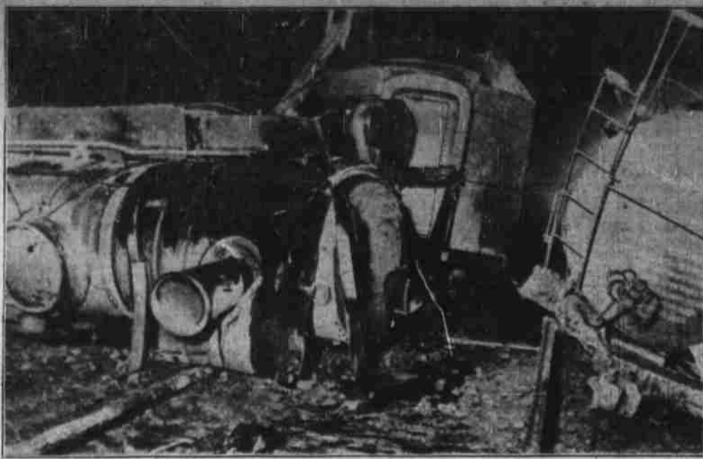
This is the way a passenger train piled up at Jacksonville, Ill., in a wreck in which the fireman and engineer were killed and several members of the crew injured. Authorities believe vandals had tampered with a switch. (Associated Press Photo)
