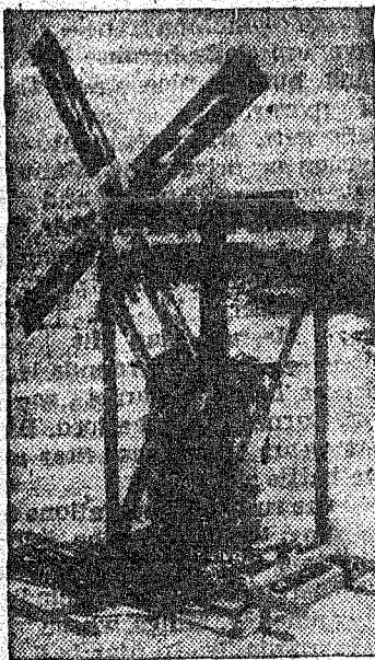
(U. S. Marine Corps Photo) Wash day is whenever the wind will blow for inventive Marines stationed in the Marshall Islands. This "windmill" washer, one of a dozen similar types in the Pacific area, permits leathernecks to pursue other duties while the wind operates the motor in the barrel and washes their clothes.
