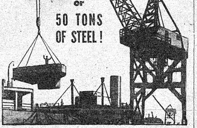
OU'RE looking at an electric "whitley" crane in action. It's placing a superstructure on the deck of a new troop transport,
