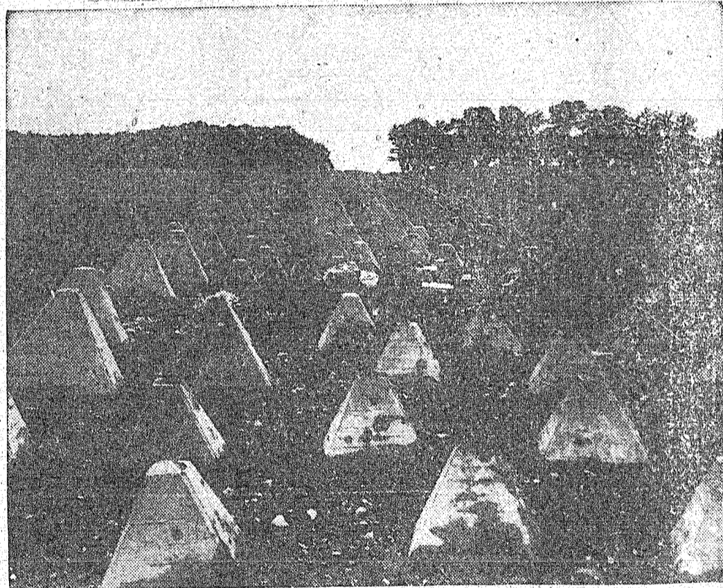
COMING THROUGH —These white objects are not tombstones, but concrete and steel obstacles placed by Nazis to delay Allies crossing Siegfried Line. Here American jeep and trailer sinks hub deep into mud to blast path through German Aachen area for oncoming American troops.
