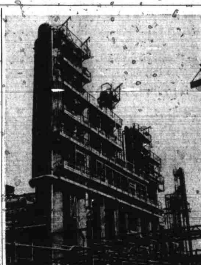
Gasoline Factory Unit—This new unit now in operation at Nederland, Tex., will produce large quantities of important component for 100-octane gasoline. It is owned by the Defense Plant Corporation and operated by Pure Oil Company.
