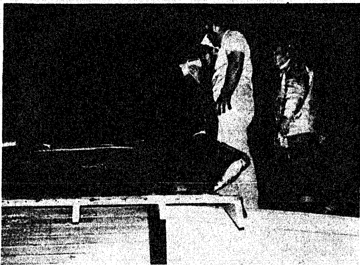
Volunteer Firemen Roddy Dean, David Huggins, and Dickie Horner look over the roof of the house at 509 S. Houston after a fire which left heavy damage to the roof and bathroom areas.
