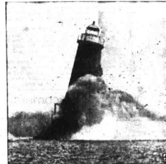
END OF A LIGHTHOUSE —Dynamite blast topples 150-year-old Bishop and Clerks Lighthouse, off Hyannisport, Mass., destroyed by Coast Guard lest it fall on fishermen.
